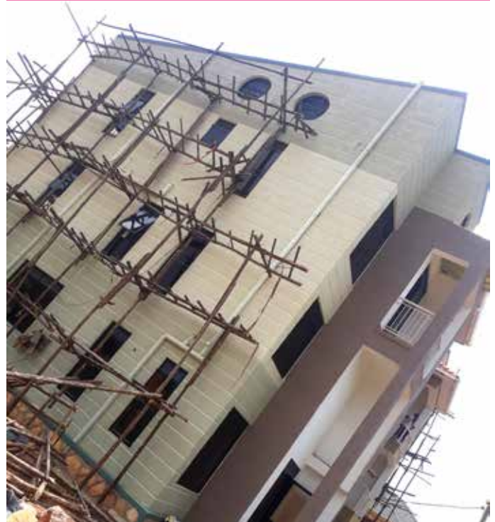
Commercial Building in Nsasa, Wakiso District
