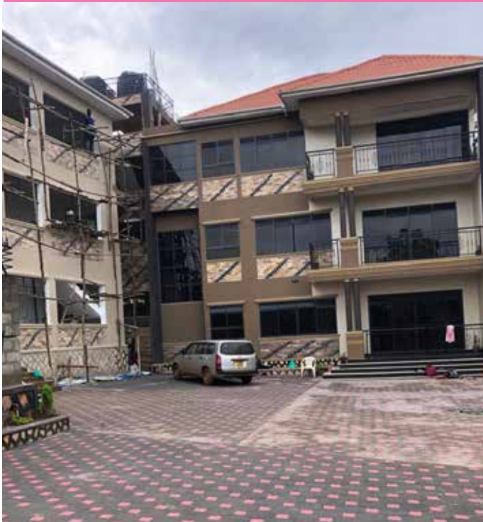
Commercial Building in Seguku, Katale, Wakiso District
