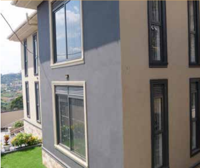
Residential Building in Bulindo, Wakiso District
