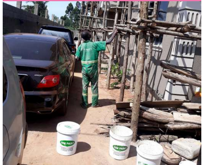
Commercial Building in Sonde, Mukono Municipal
